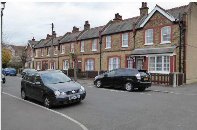
Street E east side
