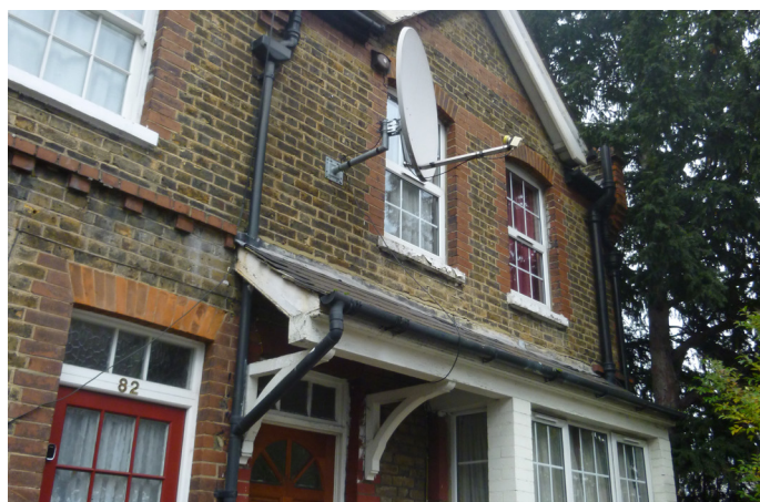
Satellite dish and replacement windows
