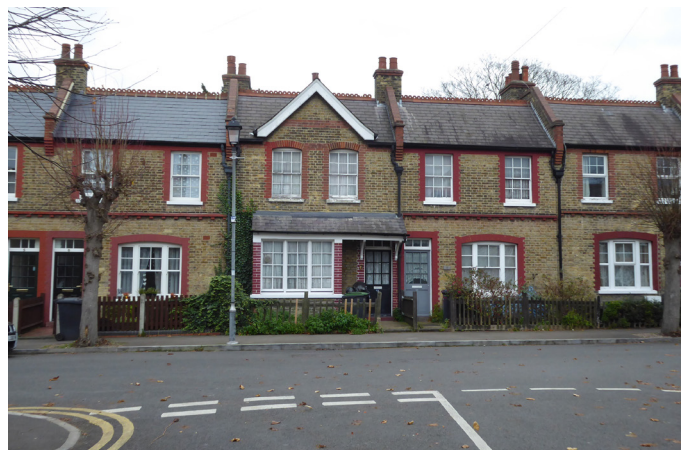
Painting of brickwork
