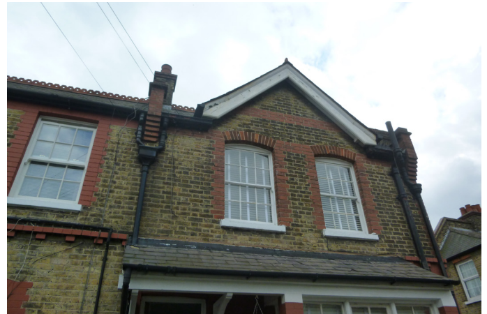
Detail of typical end-of terrace house
