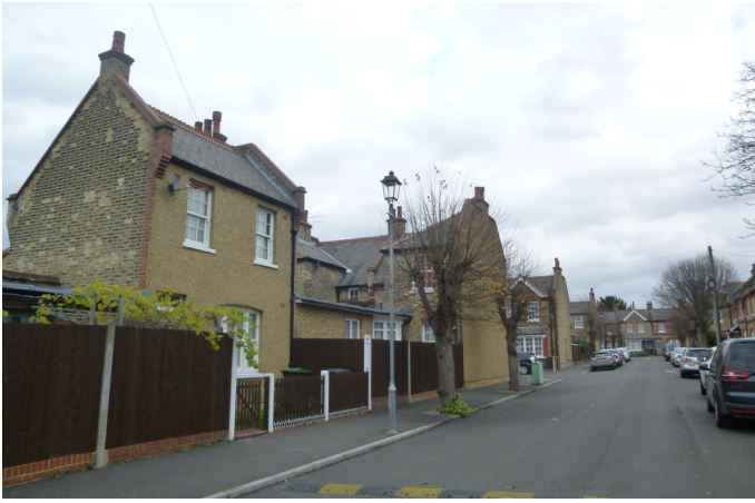
Street C north side: detached cottages, facades now rendered
